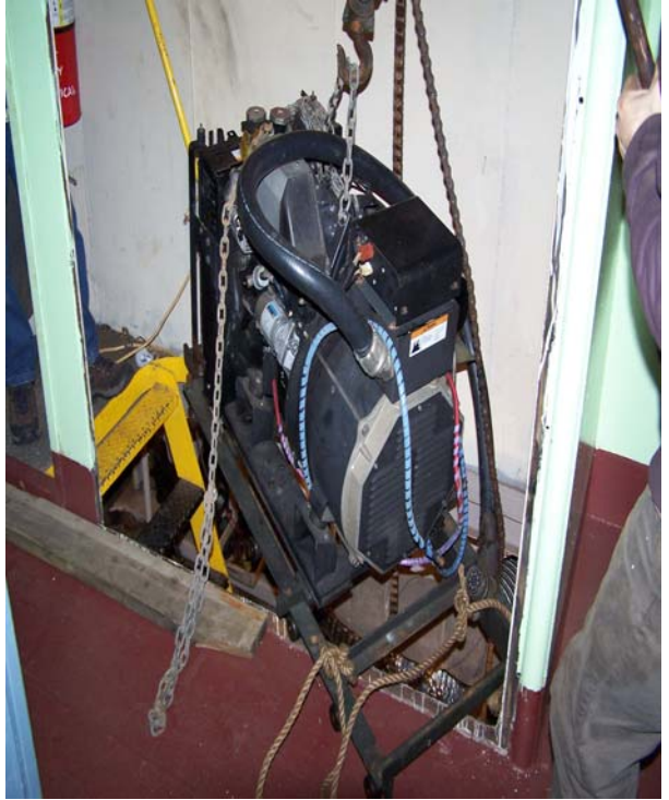
Generator positioned over the Engine room ladder well.
