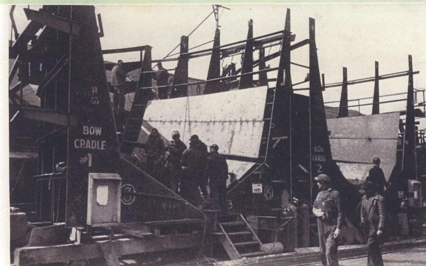
LCI'S ARE BUILT in sections which later are welded together. This shows two bow sections under construction.
